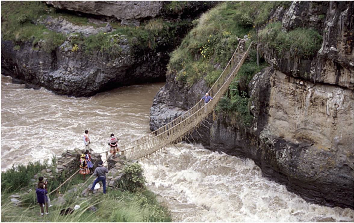
The bridge in use during the rainy season.
